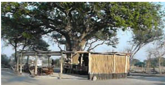
The communal area of Hanyini Research Station with kitchen, equipment storage, presentation and relaxation space.
