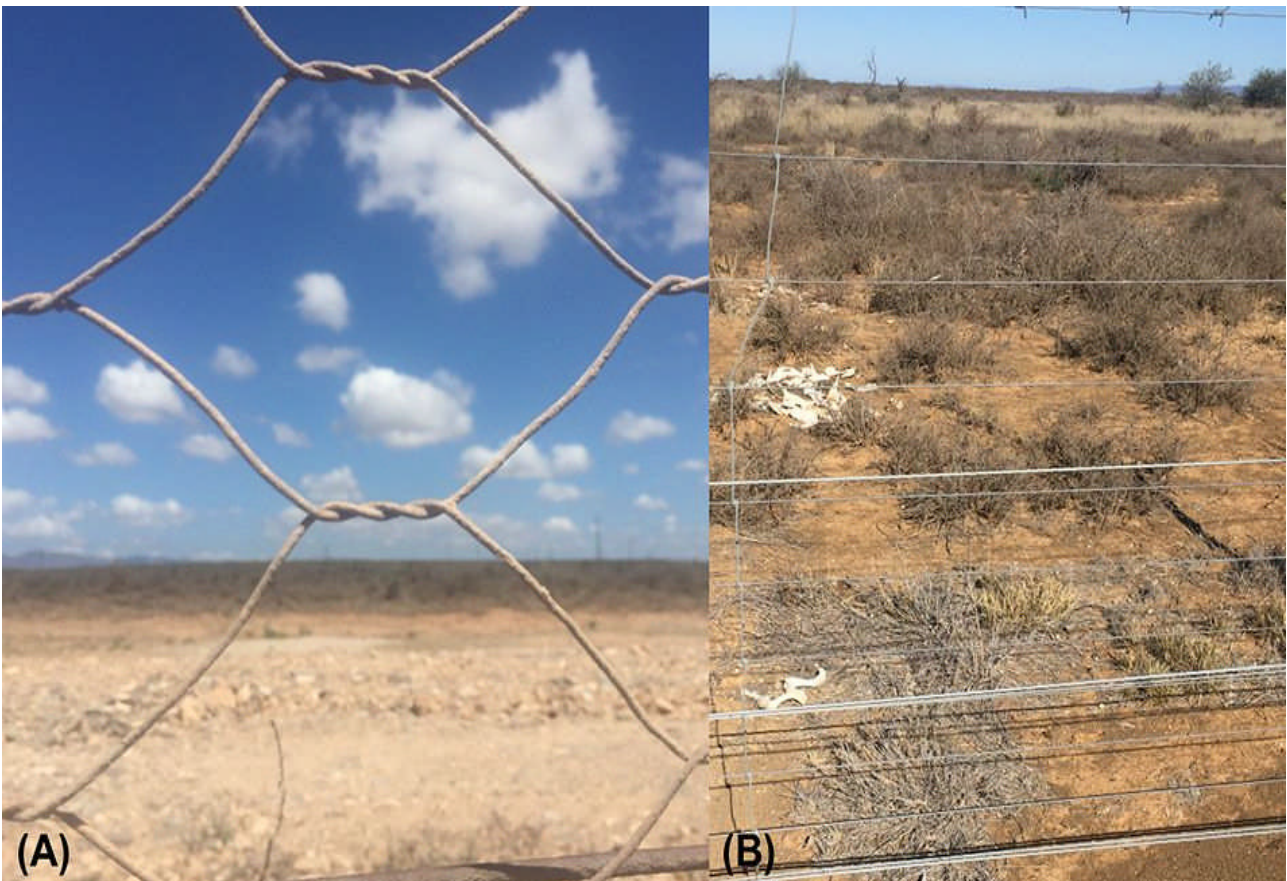
Figure 5.2a. Common fence types found in the area (A) mesh and (B) strand.
